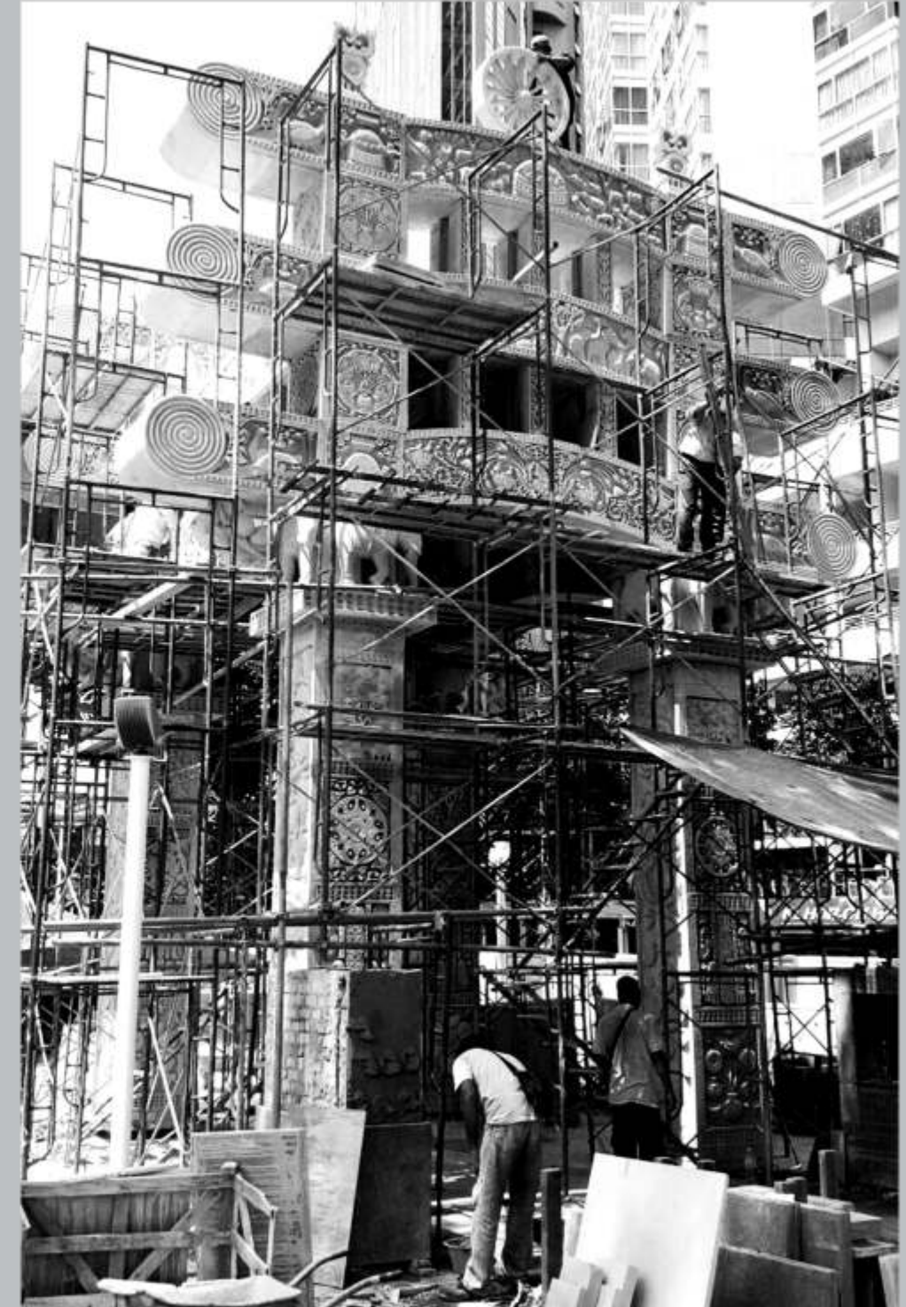
ABOVE AND LEFT | Work in Progress images of Torana Gate
