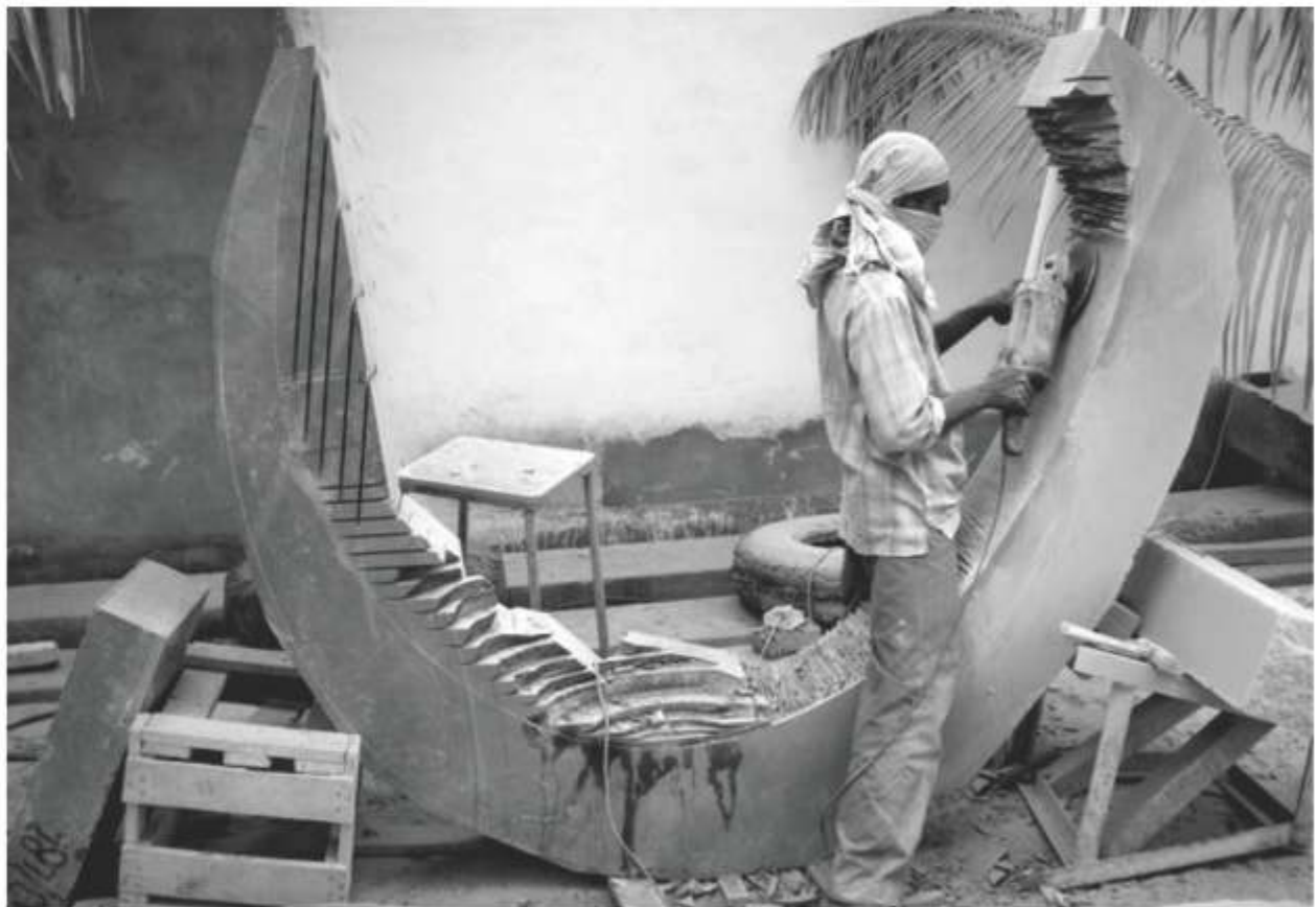
ARTWORK | Absolute Black Granite Arches, Each Carved Out of 300 mm Thick Stone and Installed on 100 mm Thick Stone Slab
