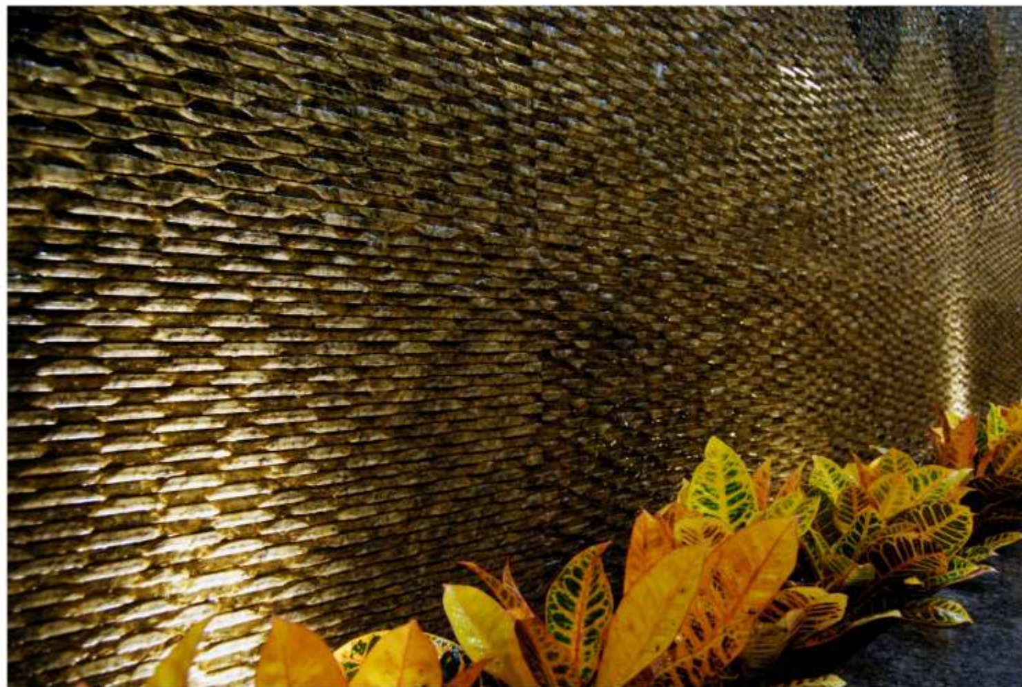
ABOVE | Internal Water Cascade Close-Up
